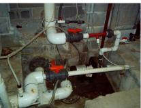
There are also smaller valves that can bleed air from filters and control the flow of chemicals into PVC lines. The same rules apply about handle direction as related to off/on.
