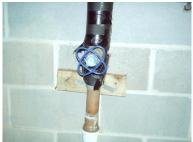
This usually turns the city (make up) fresh water supply off and on to fill the pool. Clockwise rotation of the handle closes the valve – counterclockwise rotation opens the valve and turns on the water. This is how the pool water level is controlled. Pool water level can be critical to proper operation of pool equipment.
