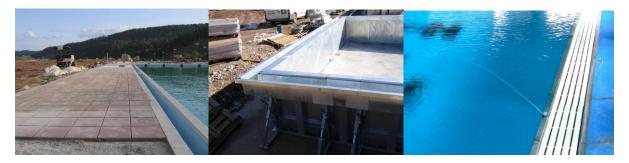
Both skimmers and gutters take surface water from the pool and get it to the filter system by piping. The larger pools usually have gutters. There are many types of gutters – some get the water off the surface more effective and efficiently than others – but their primary function is the same. Get the water to the filters.
