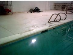
It can also be accomplished by a trough along the outer top edge of the pool around the total perimeter. These are called gutters.
